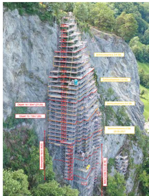
Dornisporn rock cliff monitored by Huggenberger with borehole extensometers and anchor load cells.
