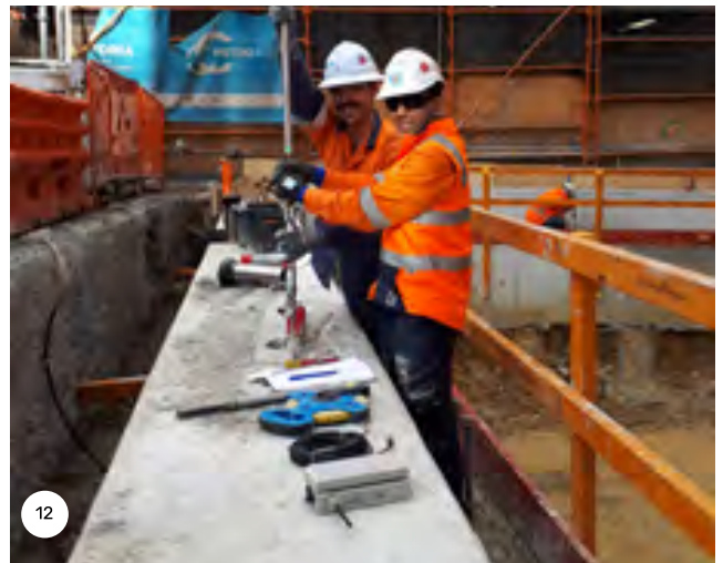
Figures 11 and 12: Personnel installing a digital logger connected to an in-place inclinometer (IPI).
