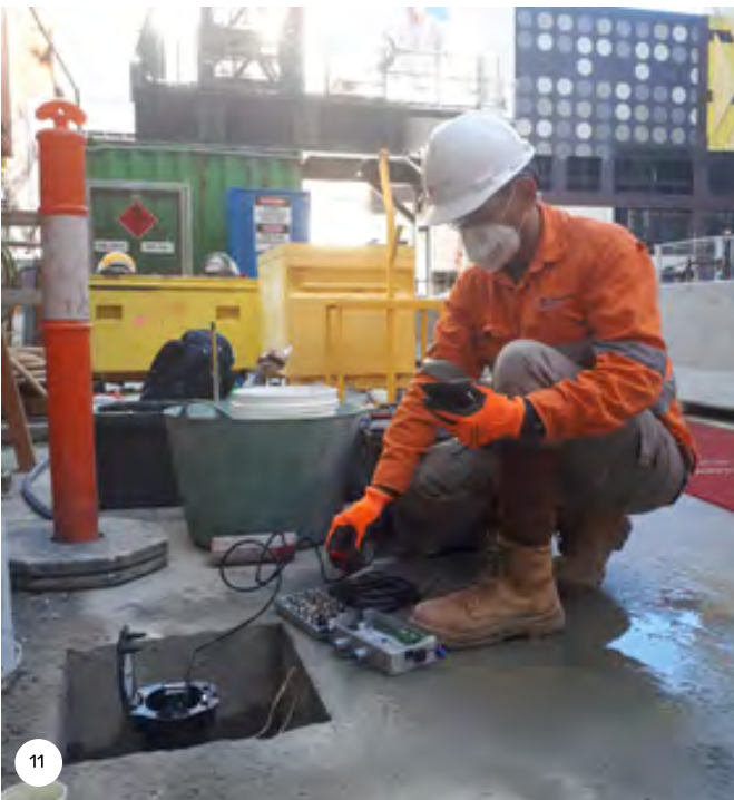
Figures 11 and 12: Personnel installing a digital logger connected to an in-place inclinometer (IPI).
