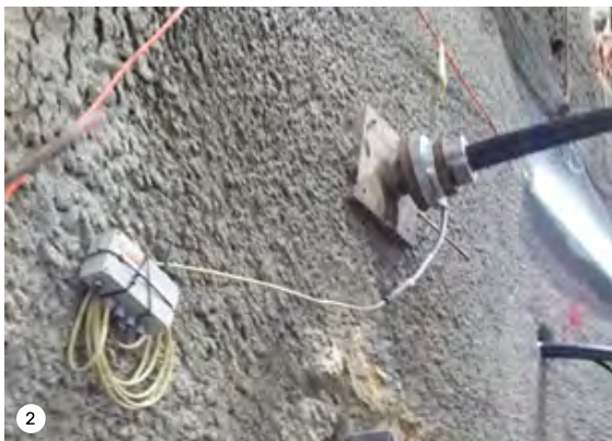
Figure 2: Anchor load cells connected to a 5-channel vibrating wire data logger.
