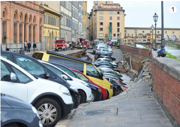
1 - The sinkhole near Ponte Vecchio, caused by a broken pipe, swallowed about 30 vehicles.
