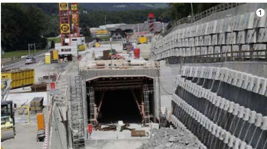
1 - The Eppenbergl Tunnel during construction
