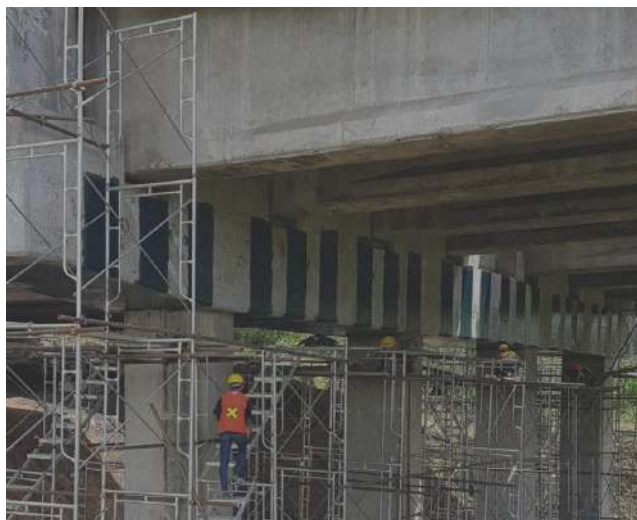
Cisomang Bridge during refurbishment
