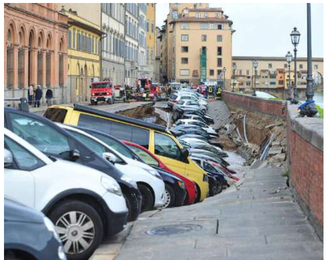
The sinkhole near Ponte Vecchio, caused by a broken pipe, swallowed about 30 vehicles
