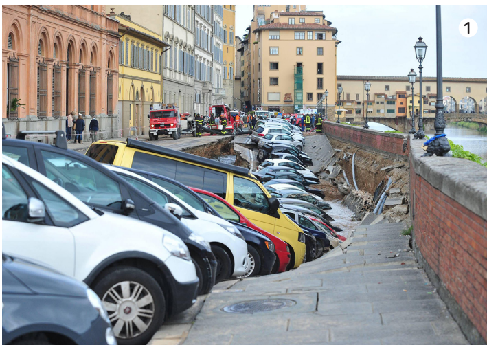
1 - The sinkhole near Ponte Vecchio, caused by a broken pipe, swallowed about 30 vehicles.
