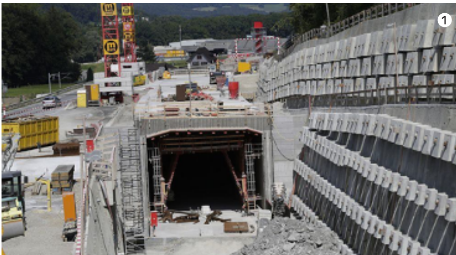
1 - The Eppenberg Tunnel during construction
