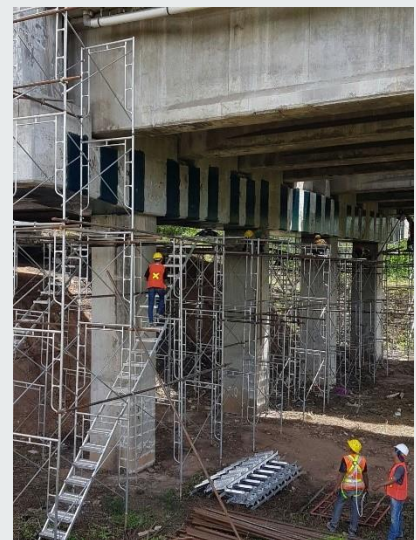
Figure 2: Cisomang Bridge during refurbishment
